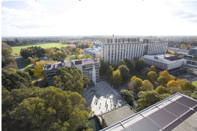
Science Department buildings, University of Canterbury
